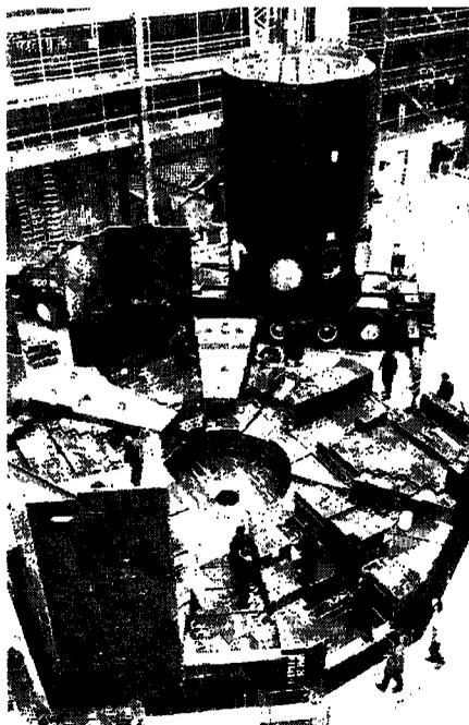
Figure 3: Deposition of the double-walled containment tank in an early phase of construction at the target station. Two - already positioned - boxes for beam tubes are also visible.
