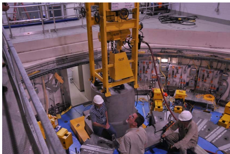
Figure 7: PBW Cask in Position for PBW Removal
