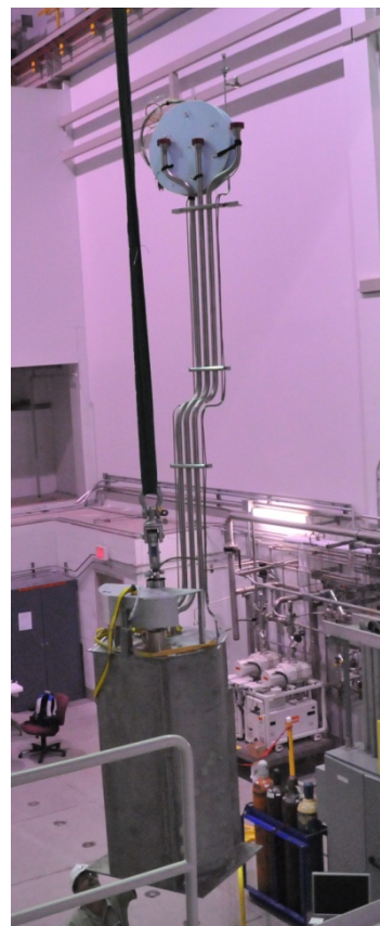
Figure 5: PBW Hoisted for Installation
