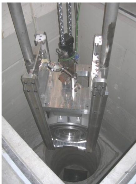
Figure 1: n_TOF new spallation target assembly being lowered in the pit.
