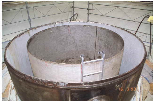
Figure 3. Steel shielding close to the center, around the inner helium tank (“helium1”) is sitting in a separate enclosure filled with a controlled nitrogen atmosphere “nitrogen1”.
