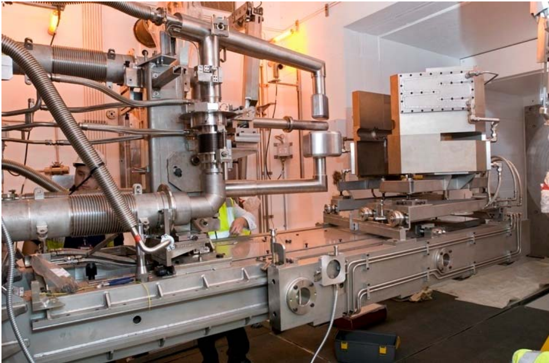
Figure 4 – ISIS TS2 TRAM in maintenance position
