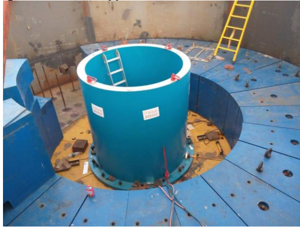
Figure19. Support skirt installment
